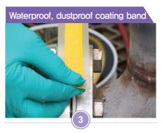
Remove the protective films on both sides of the tape and attach the tape. (Make sure to clean the area to be taped before starting work.)
